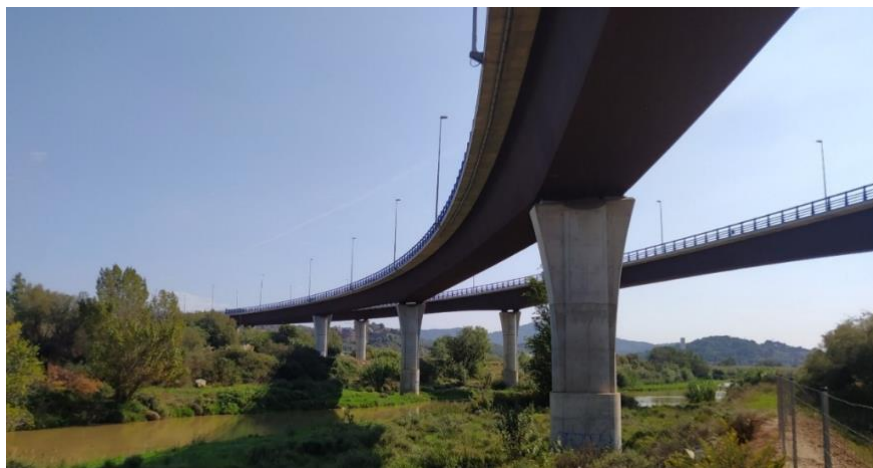
Figure 11: PR-04-B015 bridge, passing over the Llobregat river.
