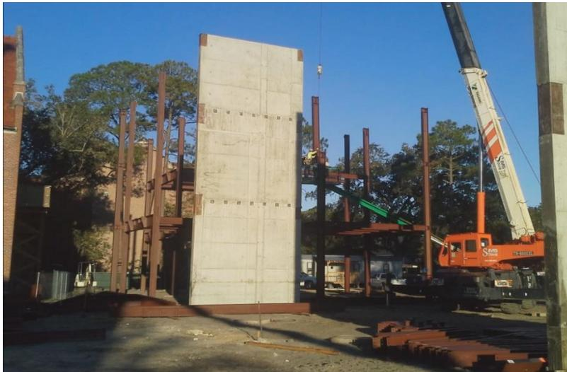
*FIG 4: Erection of structural steel*
