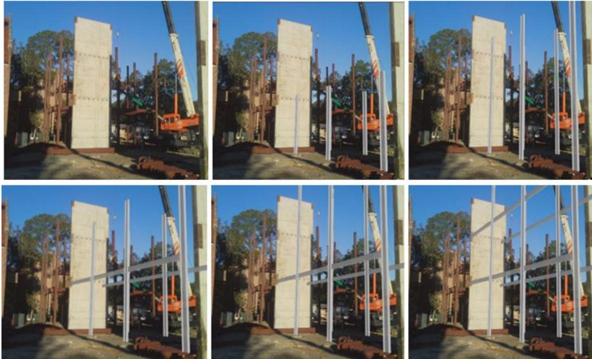
FIG. 10: Augmentation of structural steel elements over prevailing as-built jobsite conditions.
