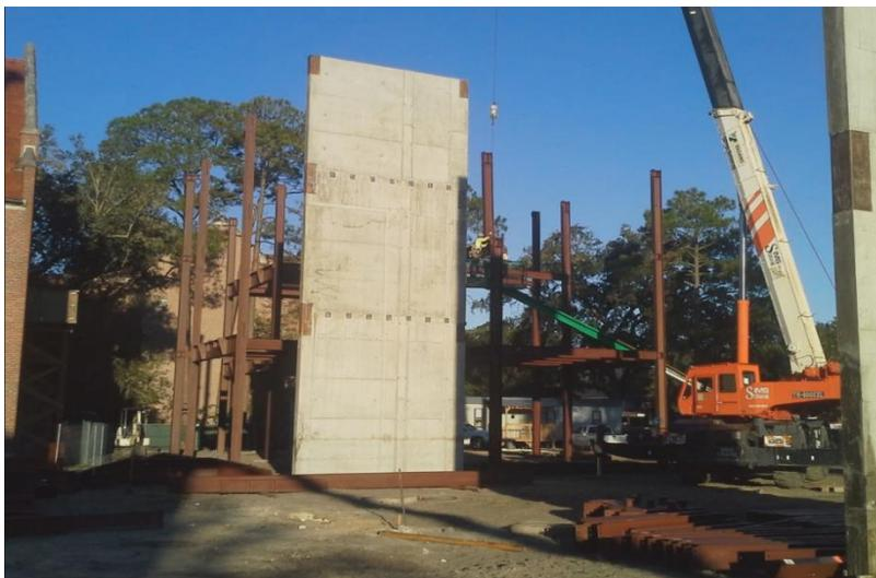
*FIG 4: Erection of structural steel*
