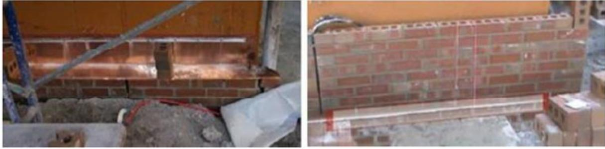
FIG. 7: Copper flashing highlighted in AR-enabled video of brick veneer installation process.
