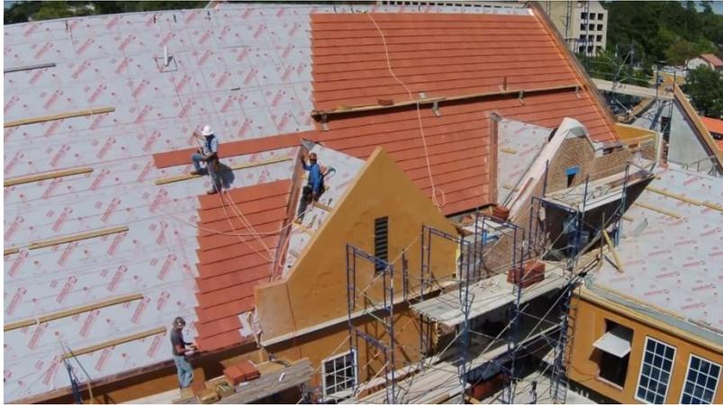
*FIG 3: Installation of clay roofing tiles.*
