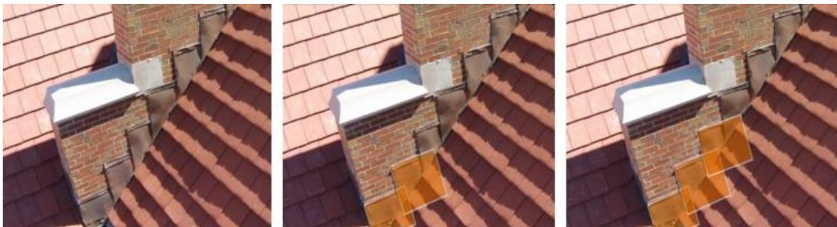
FIG. 9: Augmentation of copper flashing over prevailing as-built jobsite conditions.
