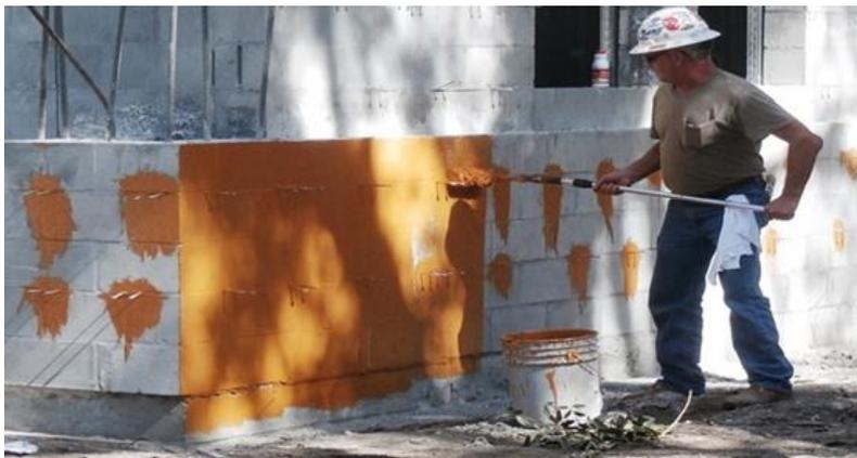
FIG 2: Installation of waterproofing on the exterior CMU wall.
