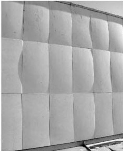
FIG. 1: Example of the clearly developed convex bowing of marble panels (Siegesmund et al. 2008).
