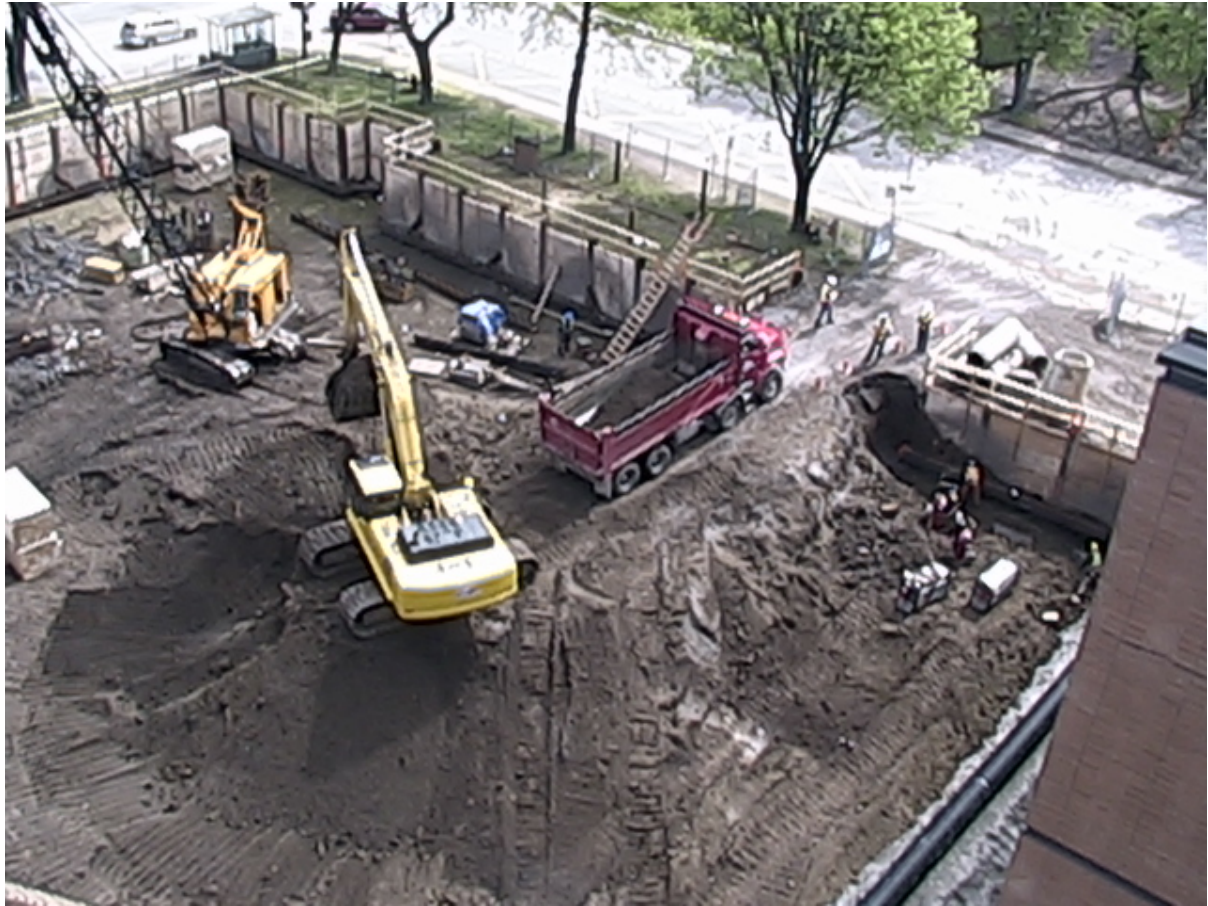
FIG. 12: Construction of CSFG building (Case Study)
