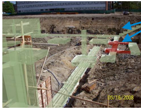
FIG. 16: The superimposed photo visualizing the component which has been misinterpreted by the carpenter foreman. Student Dining and Residence Hall project, Champaign, IL. Photograph courtesy of Turner Construction Company; Champaign, IL; used by permission.
