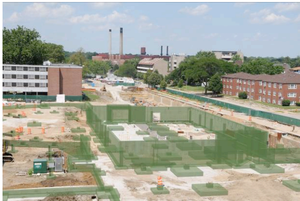
FIG. 12: The alignment of the Student Dining and Residence Hall construction project 3D model with one of the construction progress images using Golparvar-Fard et al. (2009) approach. As shown some of the foundations and foundation short walls as well as piers that are not yet constructed, are superimposed over the image. Photograph courtesy of Turner Construction Company; Champaign, IL; used by permission.
