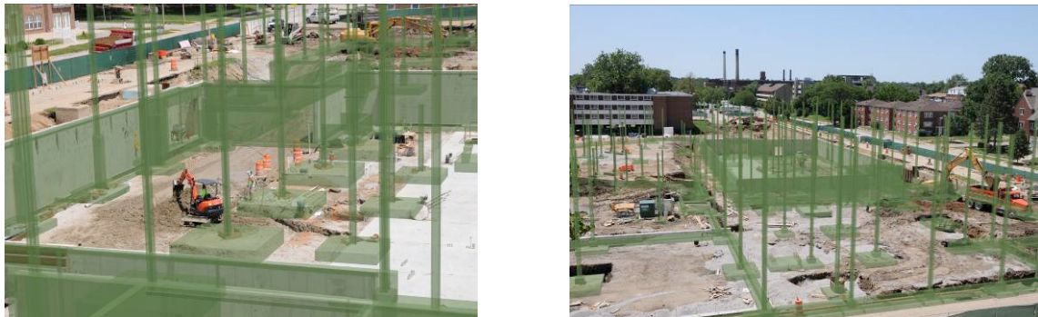
FIG. 14: The registration of images with the construction progress images. Student Dining and Residence Hall construction project in Champaign, IL. Photographs courtesy of Turner Construction Company; Champaign, IL; used by permission.
